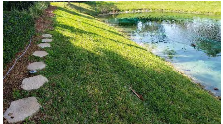
Figure 4: Lake 6 - steep slope (2.85H:1V)
