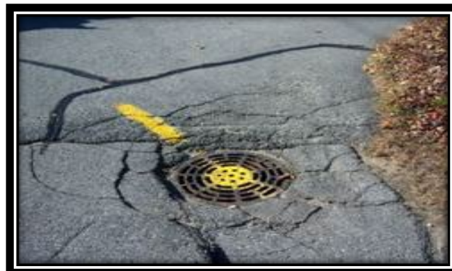
Asphalt Deterioration
