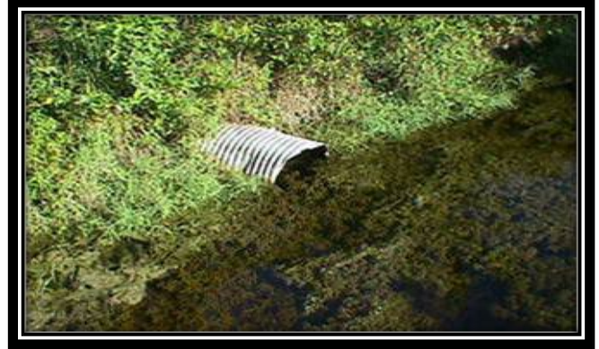
Channeling Required for Outfall
