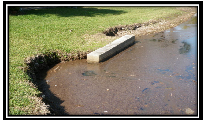
Headwall Erosion
